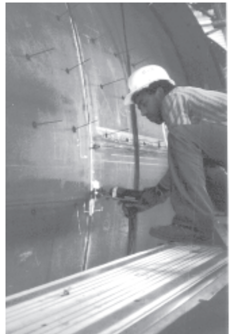
INSULATION OF A FURNACE
